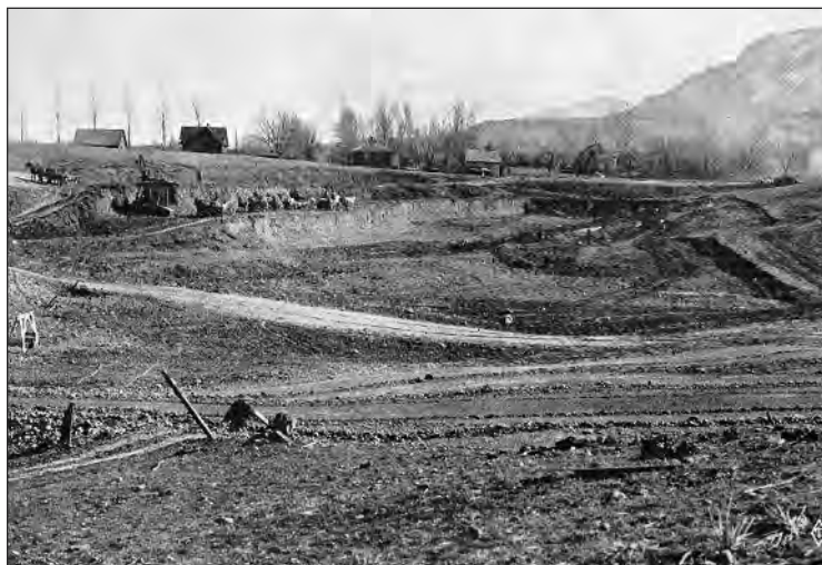
The beginning of work on the stadium in January, 1924.
