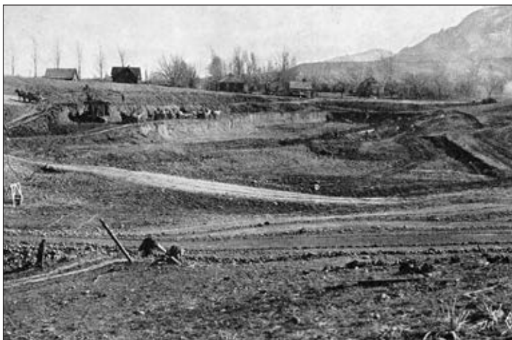
The beginning of work on the stadium in January, 1924.
